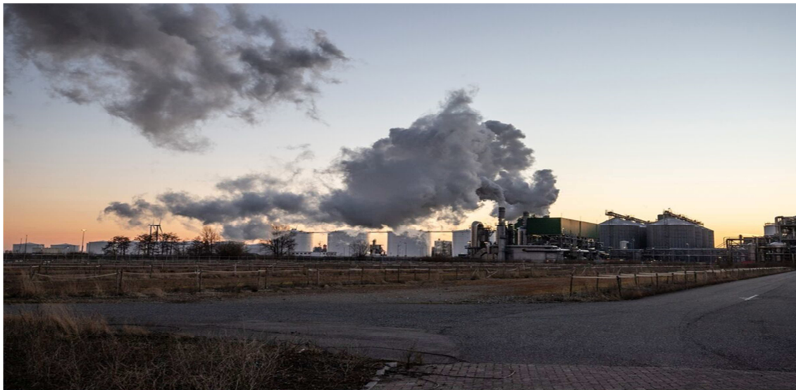
Figure 9. An Exxon Mobil Corp. refinery in Rotterdam. (Crowley, 2023; Bloomberg )
